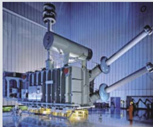
14 HVDC transformers for the long distance transmission between the three gorges hydroelectric power station and Shanghai
