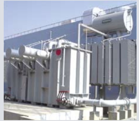
150 MVA/110 kV transformer (ONAN) with separately mounted radiator bank for BASF
